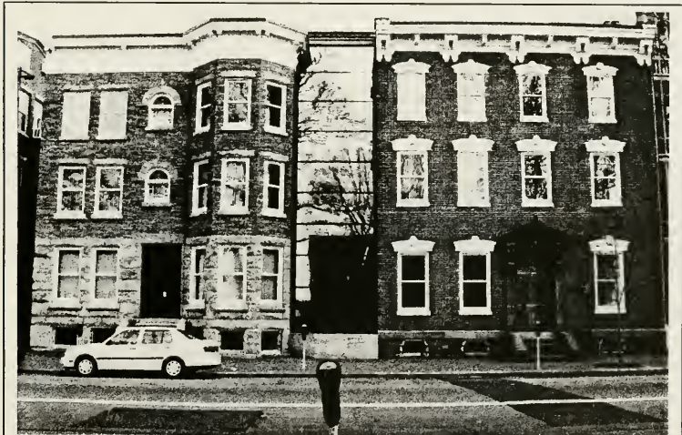
Figure 4. 186-190 West State Street Trenton, NJ. Glass enclosed stairwell connecting the two buildings. Photograph Scott Doyle.
